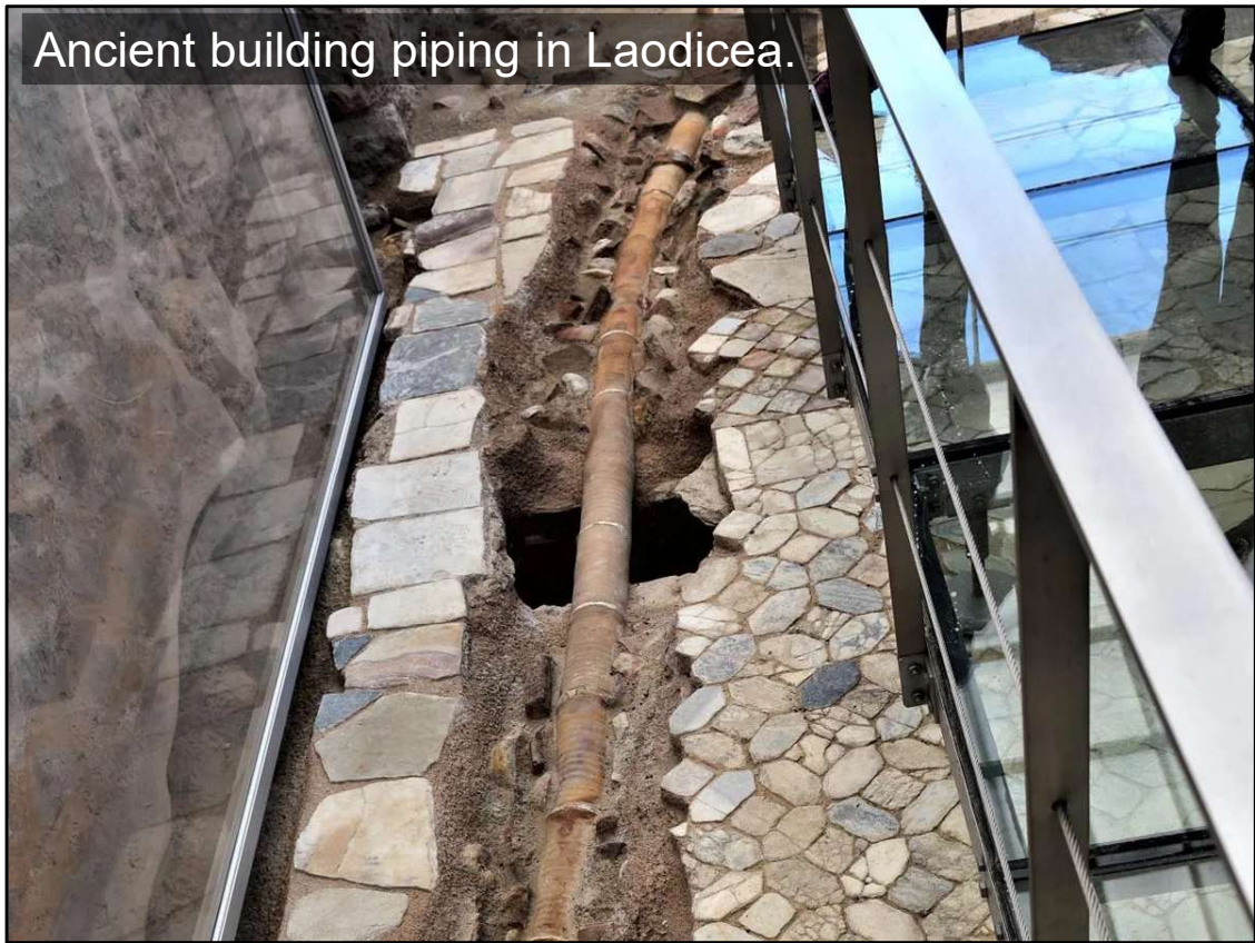
Here is some in situ distribution piping in the 4 th Century AD Laodicea Cathedral.
