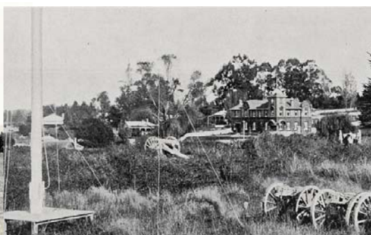
Inside the Durham Redoubt 1907
