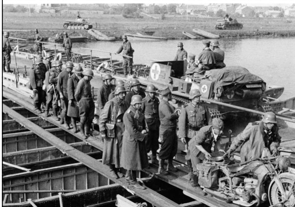
14 May 1940 1st Panzer Regiment crosses pontoon bridge over the Meuse at Floing, near Sedan
